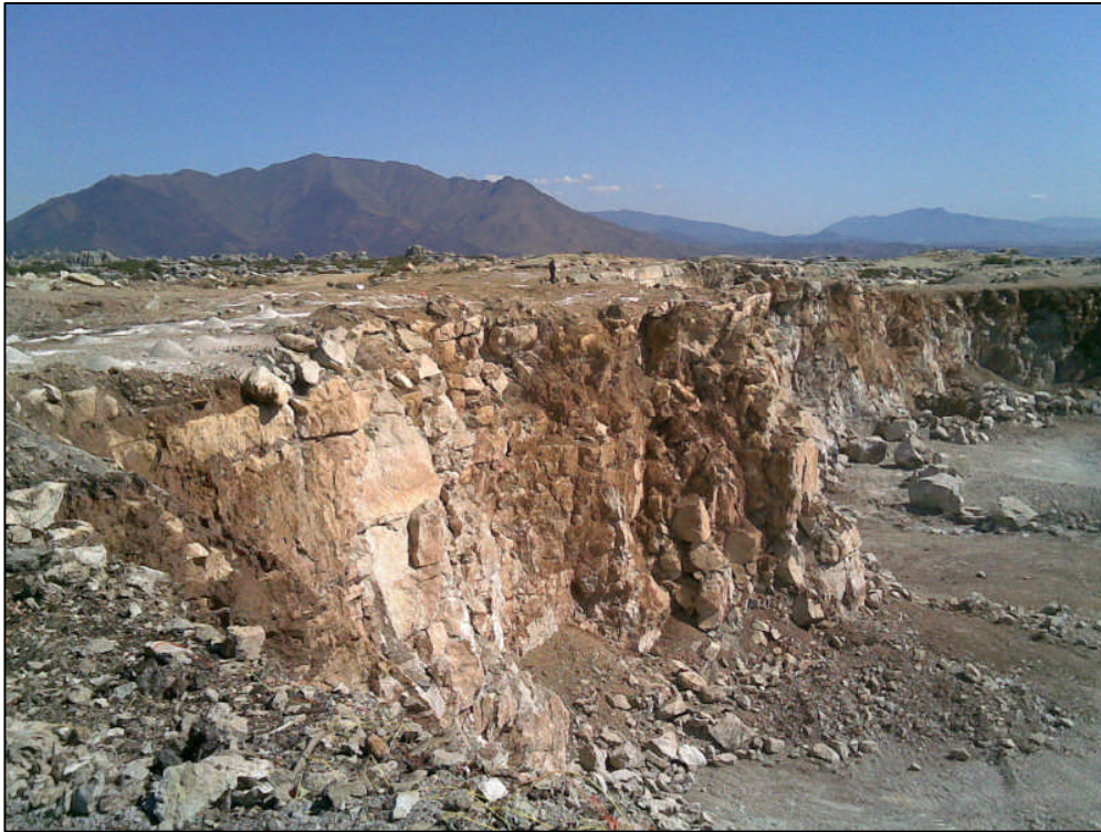
Figure 2: Overburden bench. Note the high content in clay, backfill and geology prone to be opened by adjacent blasts
